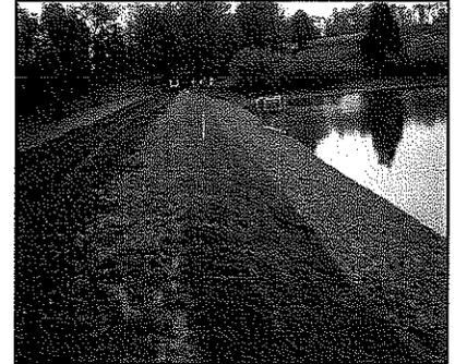
The project involved replacing the existing Corrugated Metal Pipe (CMP) riser with a new cast-in-place concrete riser structure, providing toe drain and filter diaphragm and outlet endwall with riprapped channel on downstream side, and performing minor grading and restoration of the emergency spillway crest elevation to satisfy the 100-year storm water surface requirements in the pond.
