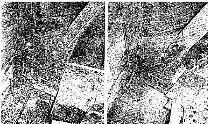
Left: Failed steel channel and riveted connection at truss. Right: Repaired connection at truss.
