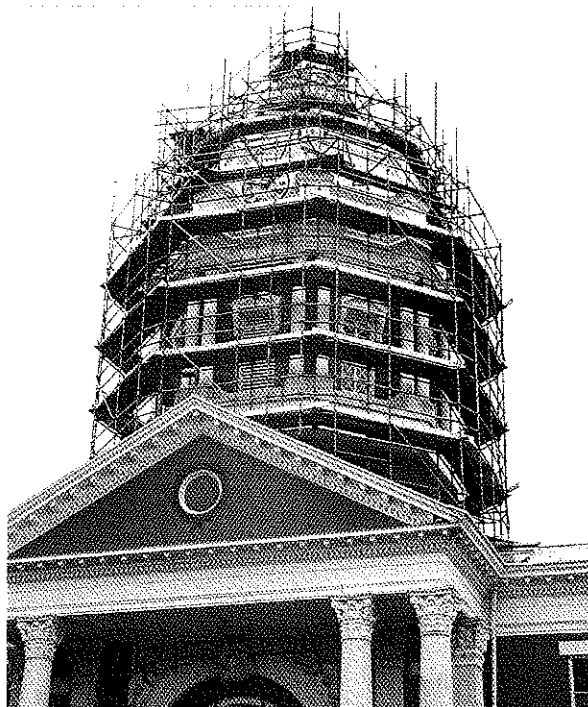
Scaffold around dome to facilitate repairs.
