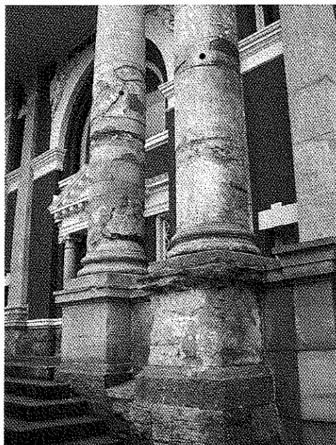
Left: Distressed sandstone columns discovered upon parging removal. Right: Restored sandstone columns and bases.
