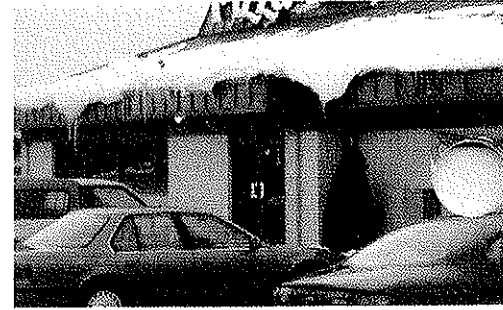
The snow above this entry door could release at any moment.
