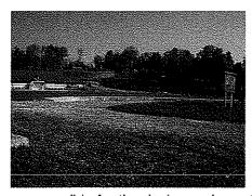
project consisted of approximately 700 tons of asphalt base course, 350 tons asphalt wearing course, crushed aggregate base course, drop inlet risers and existing concrete sidewalk removal and installation handicap ramps. G&O
