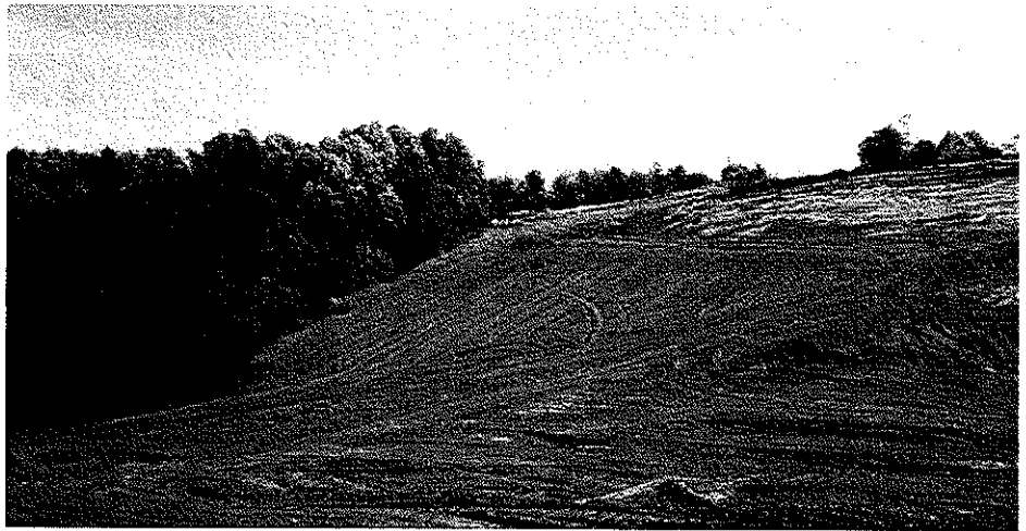
Black Dog Hollow site slope following regrading and removal of erosion features.
