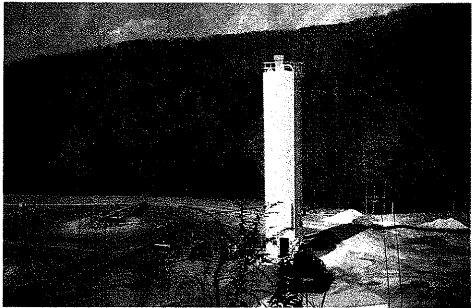
Lime storage bin, lime slaker and control unit, flash mix tank, and aeration system for treatment of AMD.
