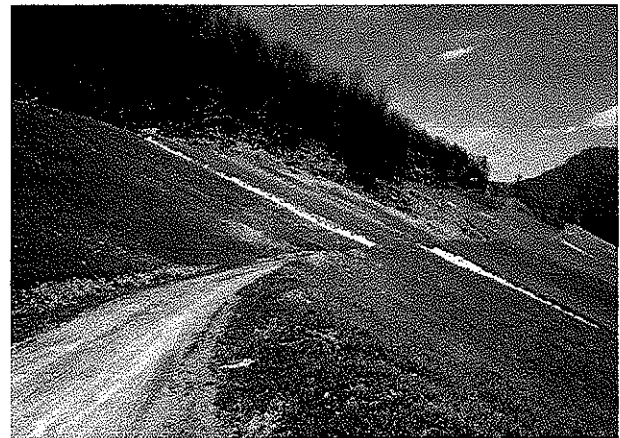
RECLAIMED NORTH REFUSE AREA
