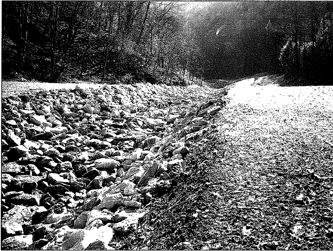
RECENTLY COMPLETED RECLAMATION OF CARTRIGHT BRANCH REFUSE PILE
