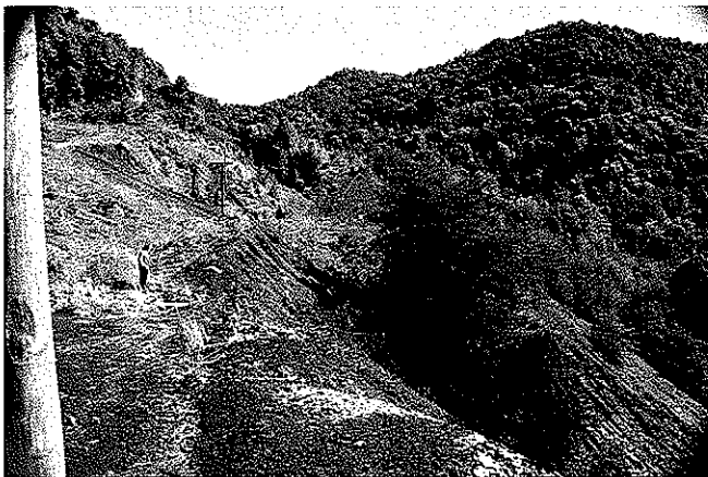
ORIGINAL NORTH REFUSE AREA
