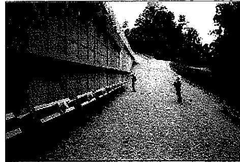
Finished wall with anchors
