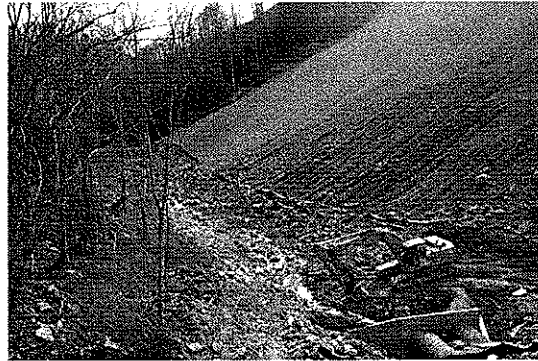
Drainage Culvert - King Coal Highway
