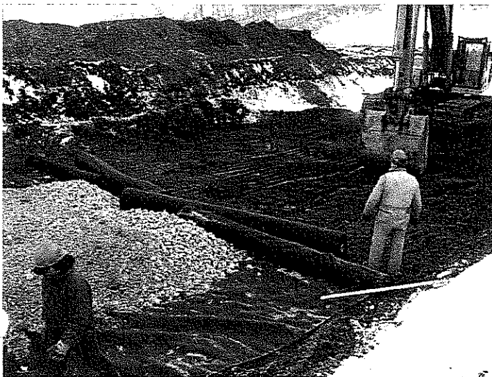
Grading and geotextile placement for internal drain construction.
