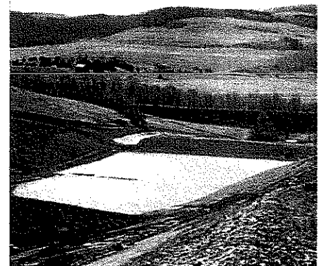
Sediment pond and lined emergency spillway channel and decant tower.
