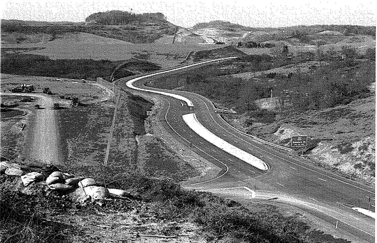
ROUTE 279, NORTH BRIDGEPORT BYPASS - COMPLETED IN 2000
