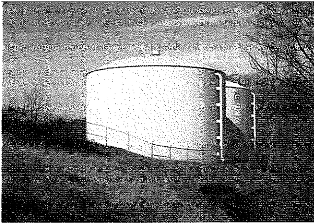
Total Project Cost = $4,400,000; Completed 1994 Two 1,000,000 Gallon Storage Tanks Part Of FBI Water Project
