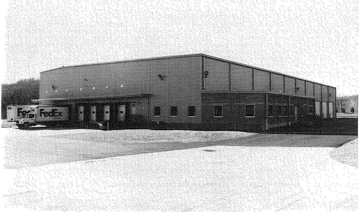
FED EX GROUND DISTRIBUTION FACILITY HARRISON COUNTY, WEST VIRGINIA COMPLETED DECEMBER 2006
