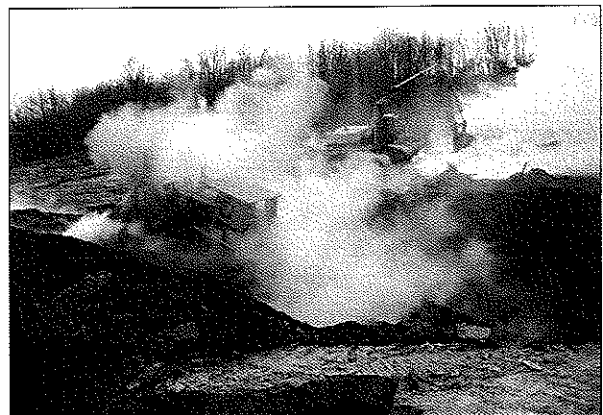
Jamison Burning Refuse Reclamation Project
