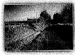
Water Resources: The Guernsey County Waterline project was considered Phase I of the northeastern waterline design for Eastern Guernsey. Wilbur Smith Associates installed 30,000 feet of 12-inch PVC SDR-14 waterline. The waterline design included a 350 foot casing bore underneath Interstate 70, and 600 feet of directional bore through Old Washington. WSA also
