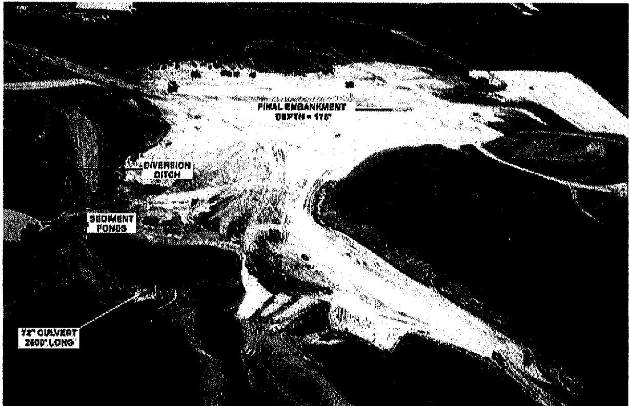
BENEDUM AIRPORT RUNWAY EXTENSION PROJECT - 1999
