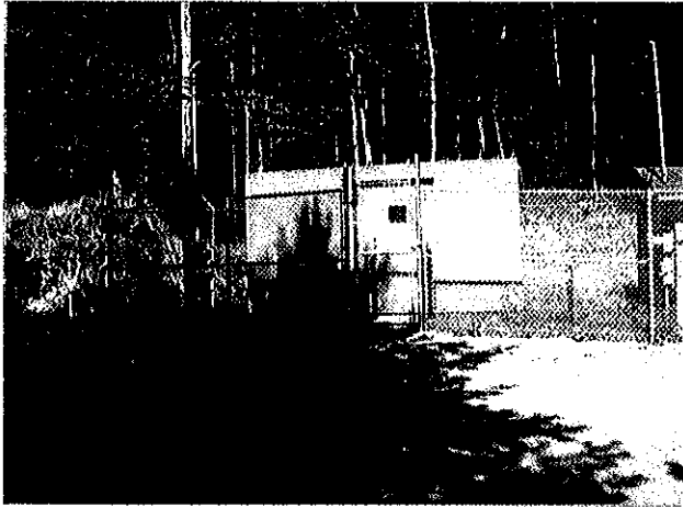
150 GPM Little Sand Run Booster Station
