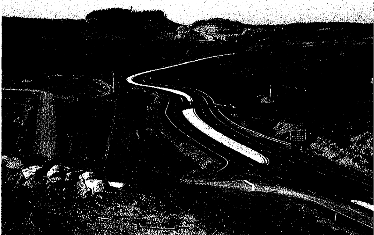
ROUTE 279, NORTH BRIDGEPORT BYPASS - COMPLETED IN 2000
