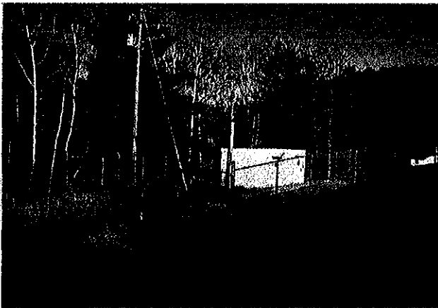
50 GPM Wilsonstown Booster Station
