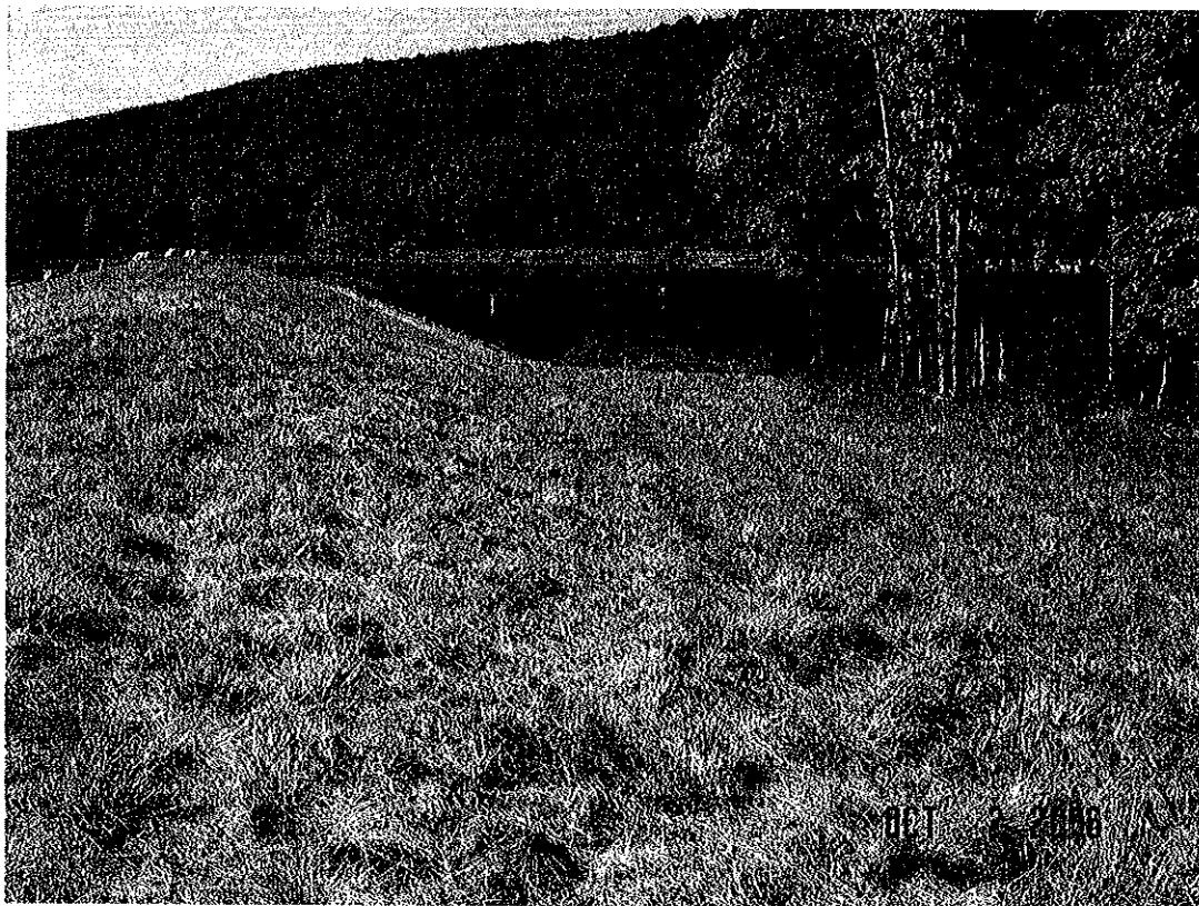
WARDEN LAKE DAM MODIFICATION, HARDY CO., WV
