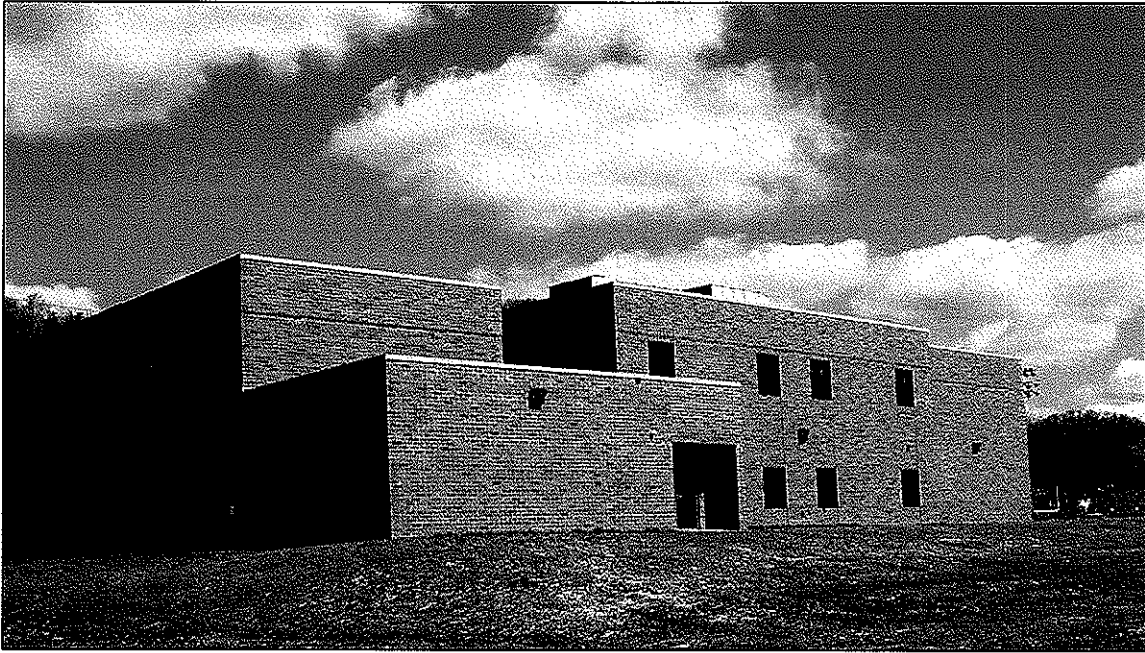
Classroom Wing Addition
