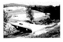
County Route 18/20 and the new Tyler County School Bridge over Point Pleasant Creek was constructed as an access to the new Tyler County Middle / High School. The bridge is a 3-span (32 ft - 40 ft - 32 ft) structure utilizing AASHTO M270 W18 beams.
