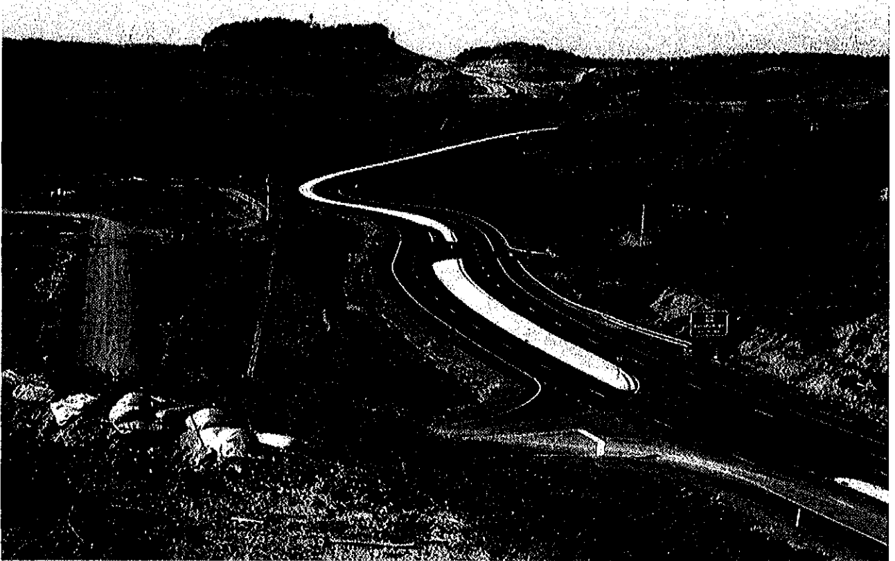
Route 279, North Bridgeport Bypass – Completed In 2000
