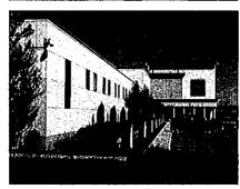
The exterior window-wall construction in the existing building was replaced with new energy efficient windows and a solid insulated EIFS clad wall system.
