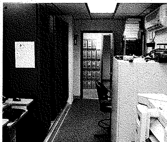
Figure 30, The Bureau's Class III Data Center showing primary server racks (left), spare systems and servers (back), auxiliary air handlers (top right), external battery pack (center right) and UPS (bottom right)
