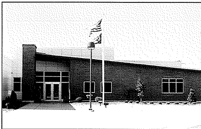
Engineering Training Center - Zane State College (formerly Muskingum Area Technical College)
