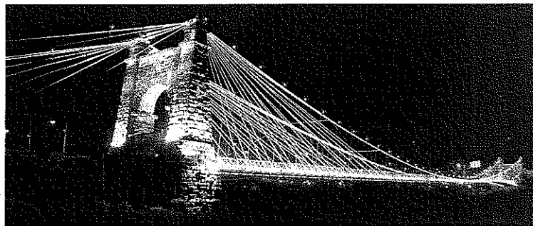
Wheeling Suspension Bridge
