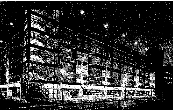
First Avenue Garage, Pittsburgh Parking Authority
