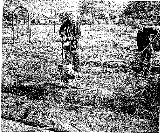
Start with a base of compacted aggregate
