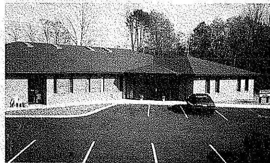
Valley Mental Health Clinic's Substance Abuse and Recovery Center features sleeping quarters for in-patient residents and staff
