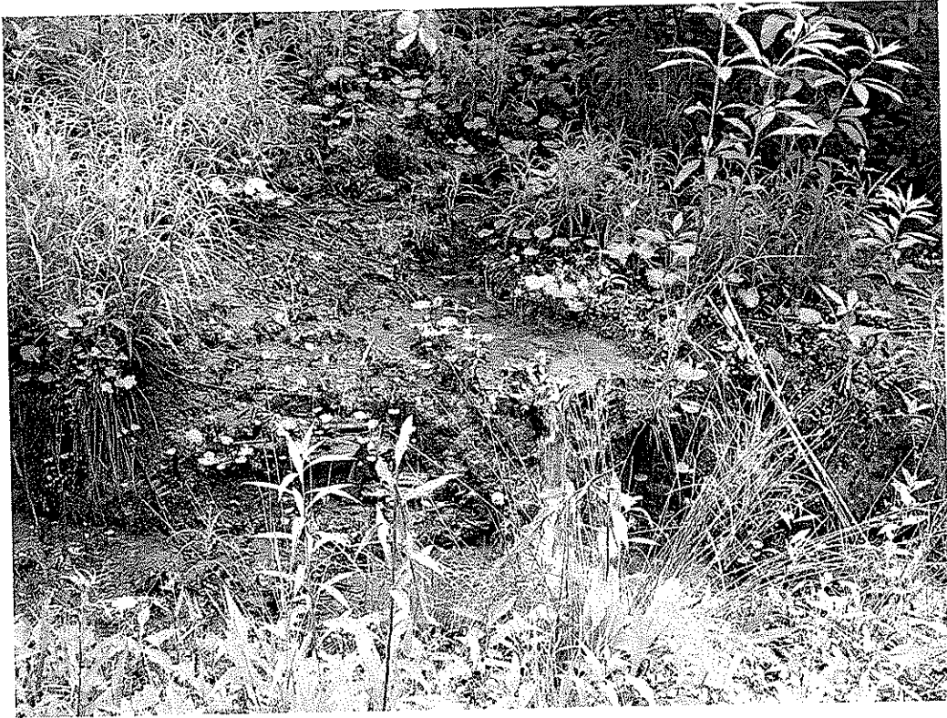
Drainage area below one of the portals
