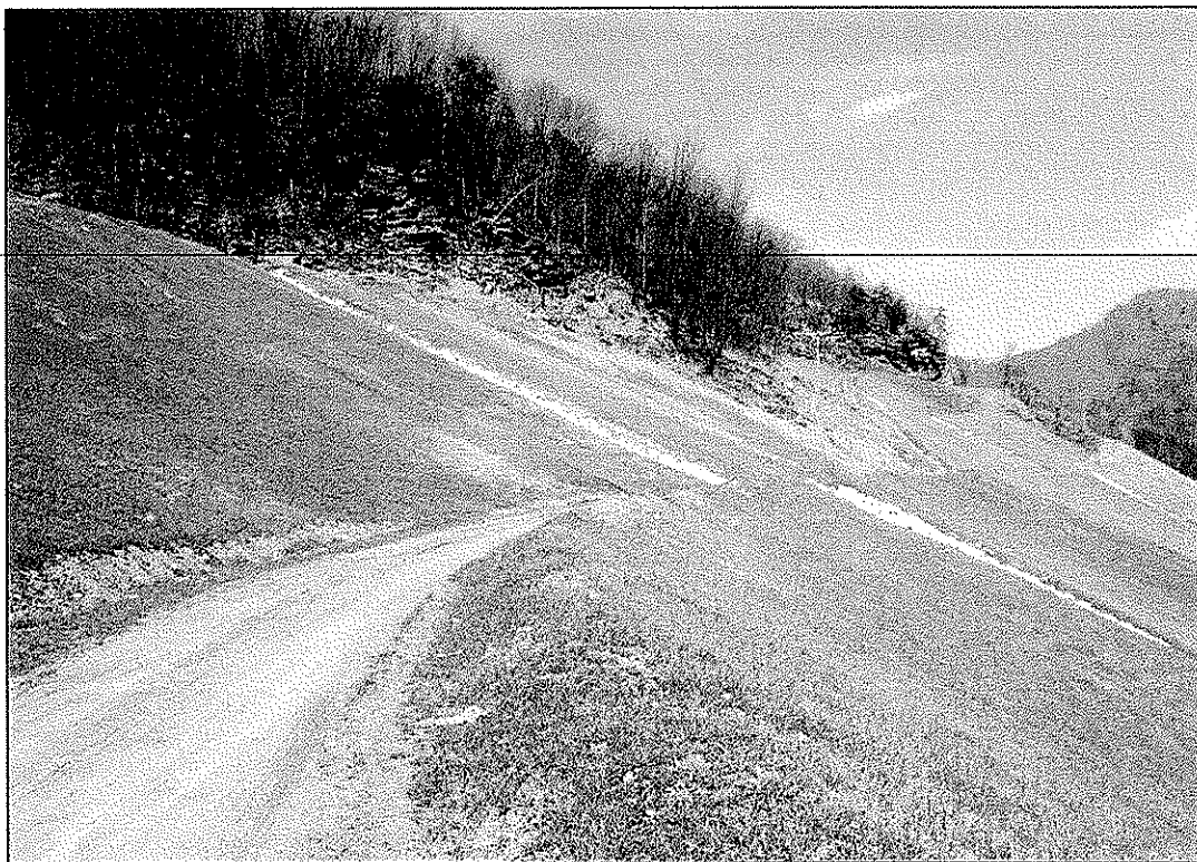
CANEBRAKE COMPLEX — McDOWELL COUNTY RECLAIMED REFUSE PILE
