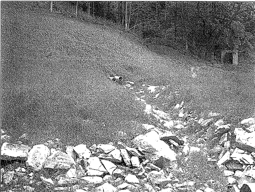
PORTAL NO. 3 WET SEAL OUTLETS AND RIPRAP COLLECTION CHANNEL
