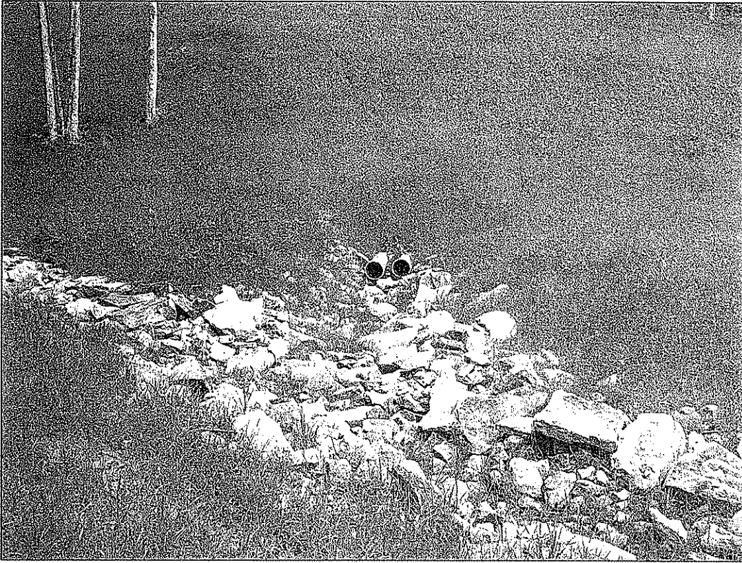
PORTAL NO. 2 WET SEAL OUTLETS AND RIPRAP COLLECTION CHANNEL
