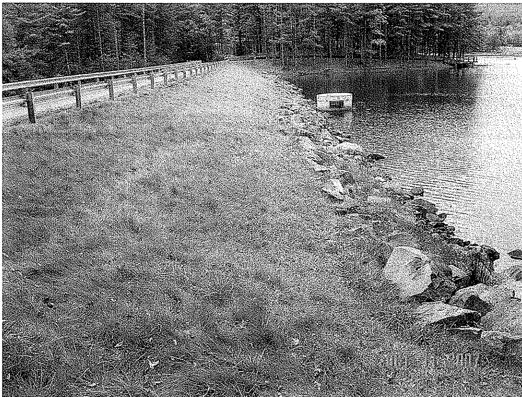
MONCOVE DAM MODIFICATION, MONROE CO., WV
