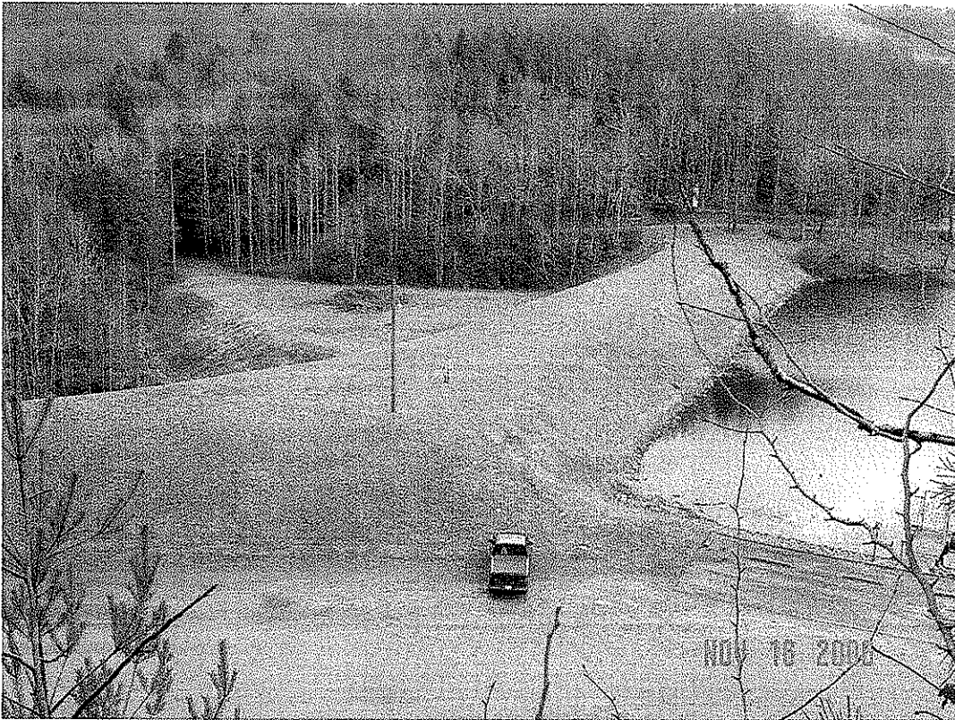
PLUM ORCHARD DAM MODIFICATION, FAYETTE CO., WV
