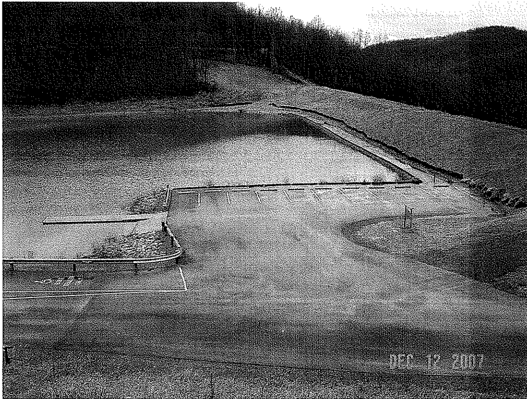
BAILEY DAM MODIFICATION, MONONGALIA CO., WV
