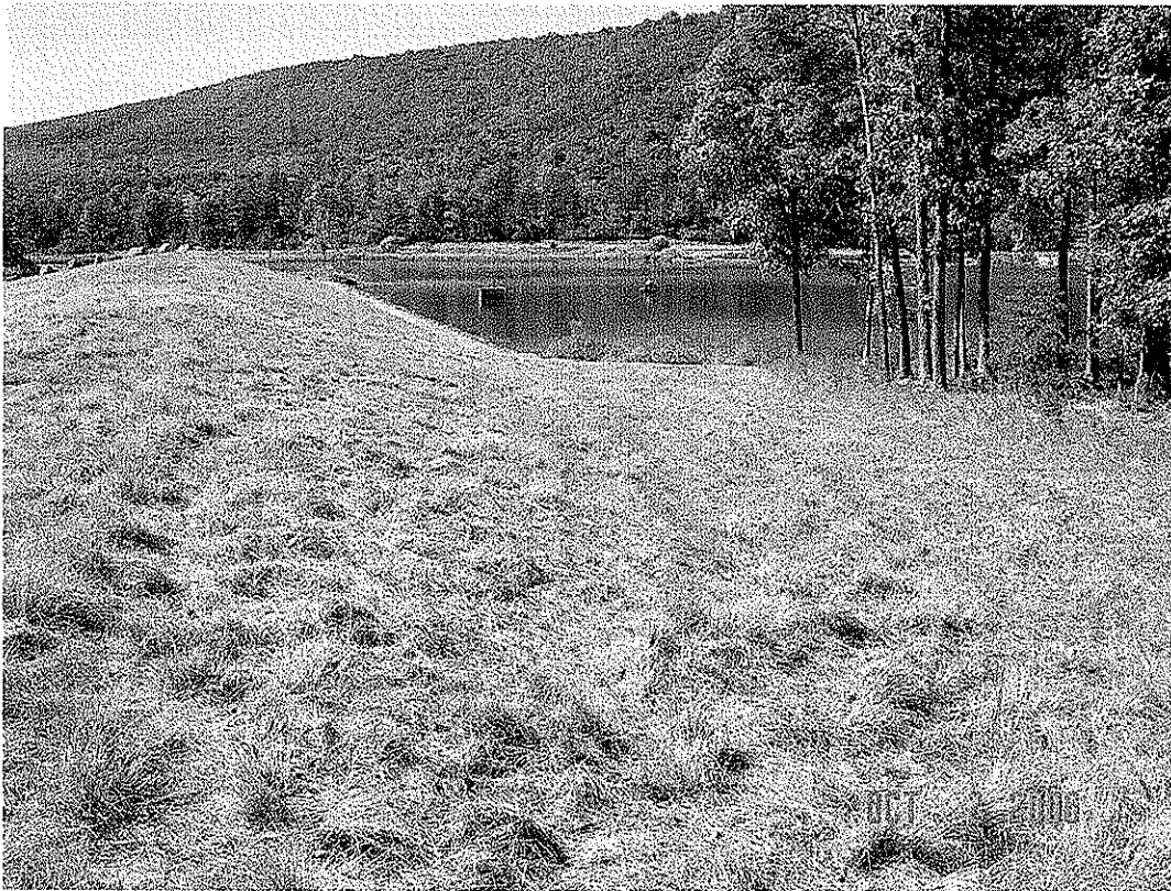
WARDEN LAKE DAM MODIFICATION, HARDY CO., WV
