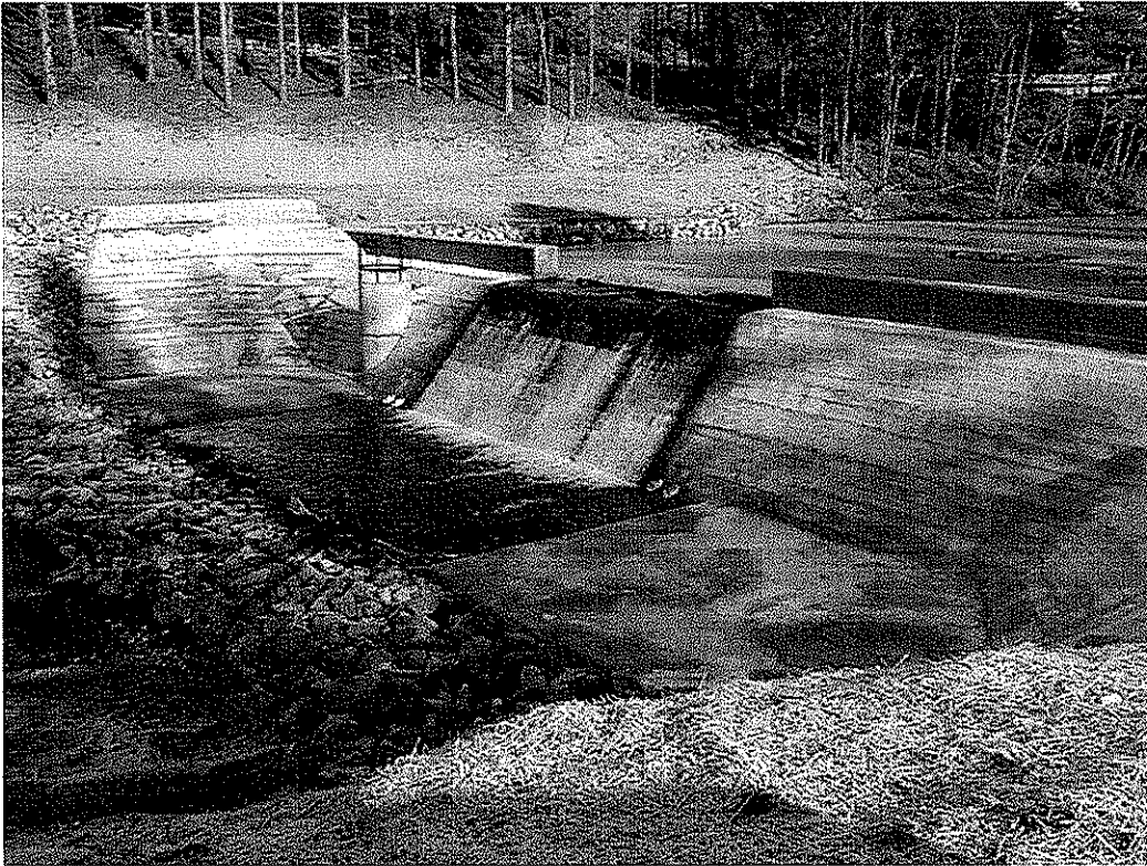
THOMAS DAM MODIFICATION, THOMAS, WV
