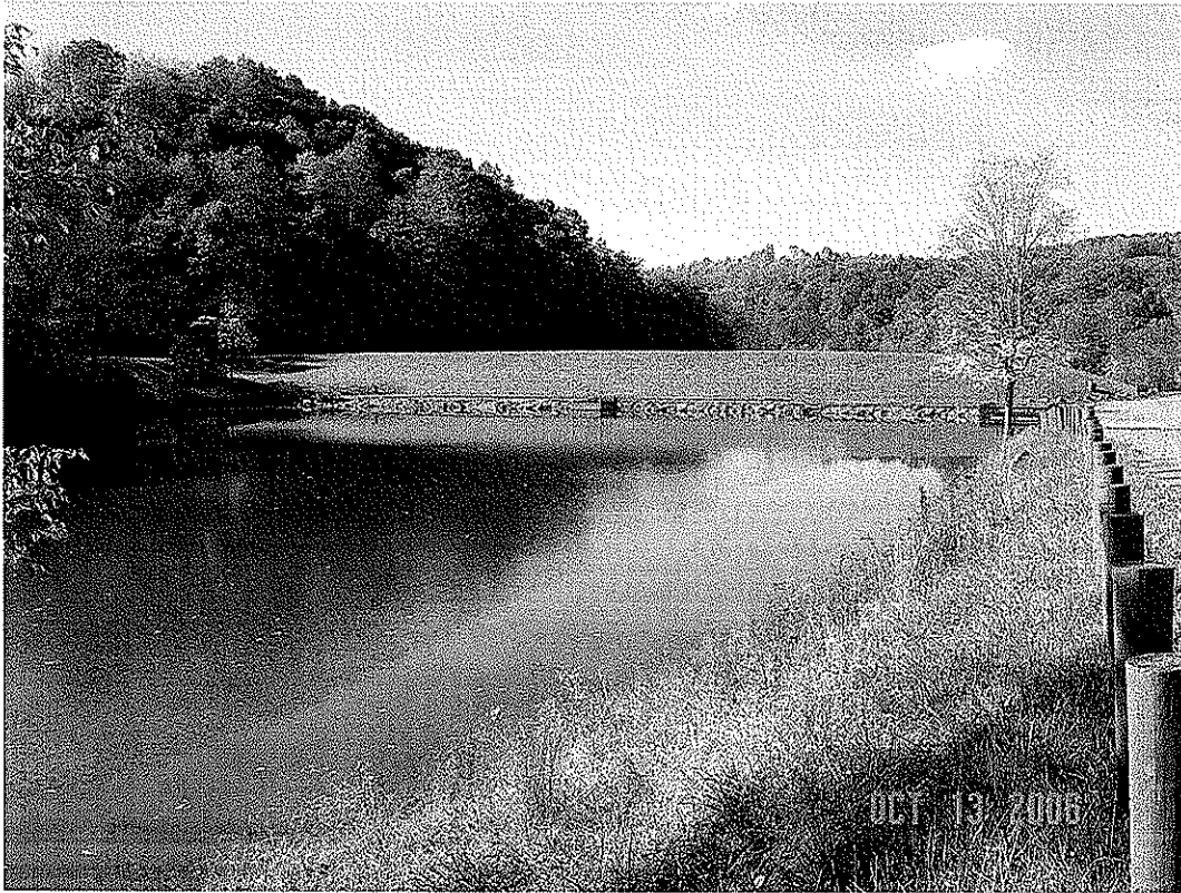
JIMMY LEWIS DAM MODIFICATION, MERCER CO., WV
