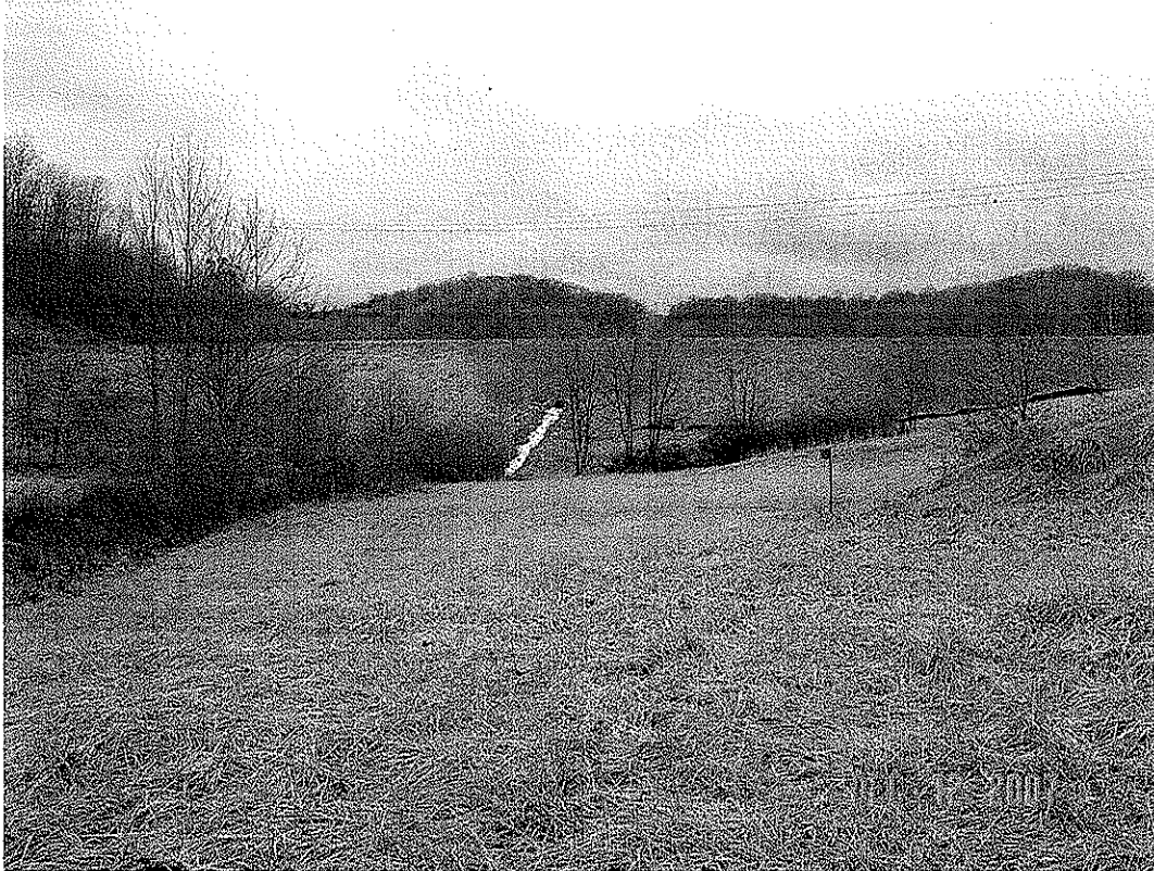
LEMLEY DAM MODIFICATION, MONONGALIA CO., WV
