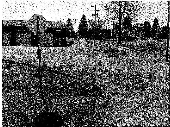
New Storm Drains and Catch Basins
