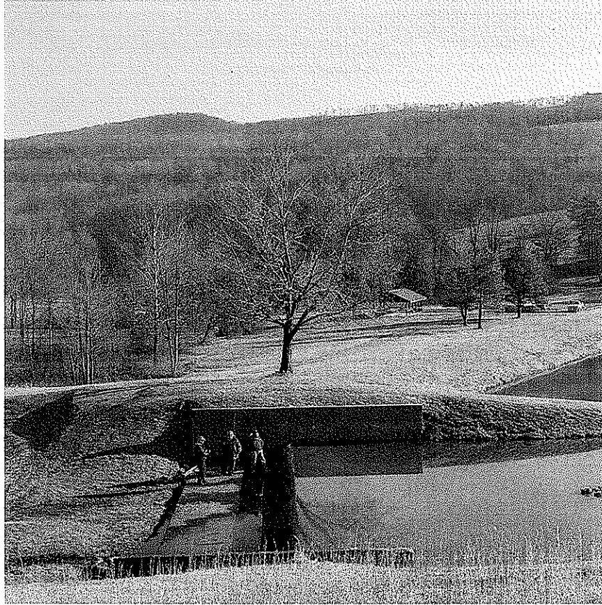
BELINGTON DAM MODIFICATION, BELINGTON, WV
