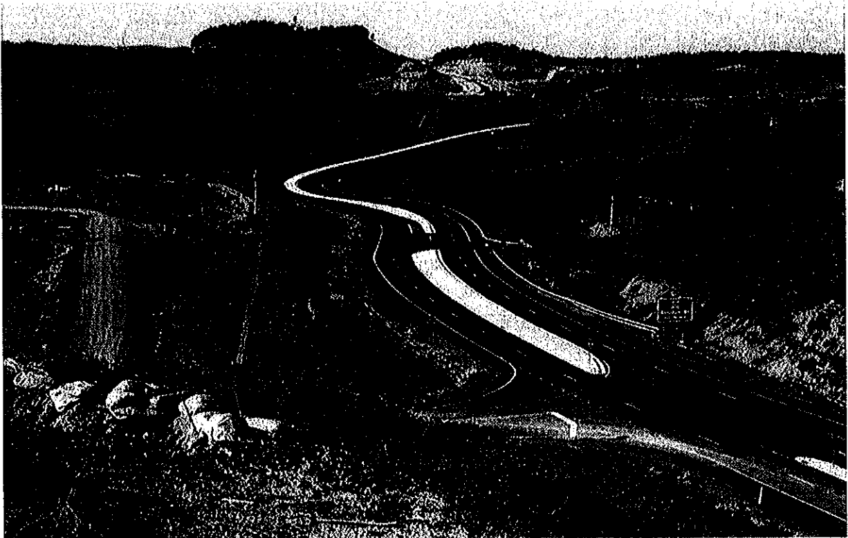
ROUTE 279, NORTH BRIDGEPORT BYPASS - COMPLETED IN 2000
