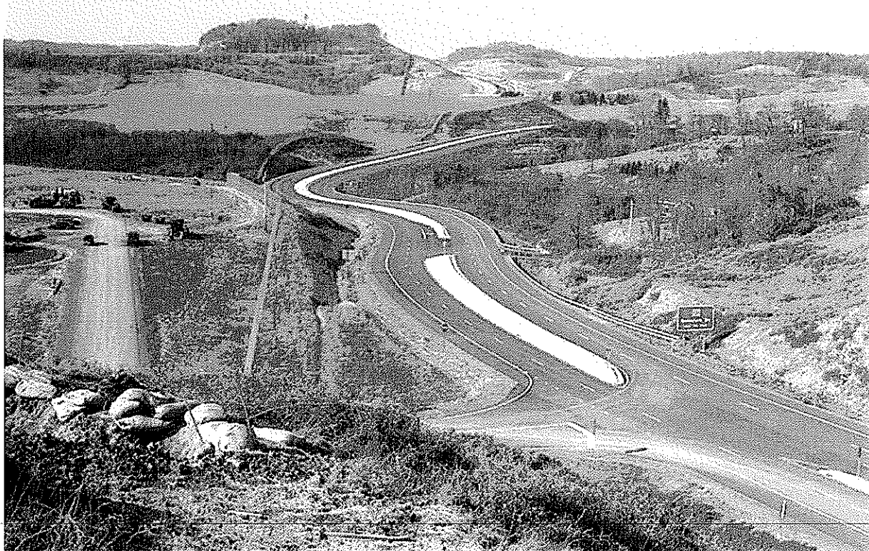
ROUTE 279, NORTH BRIDGEPORT BYPASS - COMPLETED IN 2000
