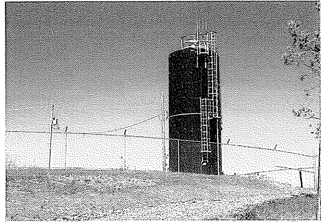
43,000 Gallon Salem Ridge Water Storage Tank
