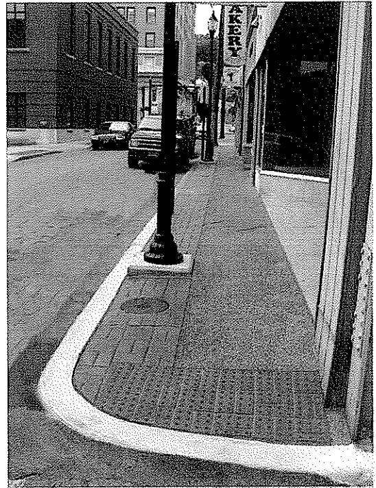
West Side of South Third Street
