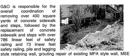
style retaining wall, and the replacement of 76 square yards of asphalt along High Street. G&O provided the planning, detailed design, specifications, cost estimates, construction bid documents, and construction engineering and inspection.
