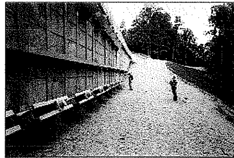
Finished wall with anchors
