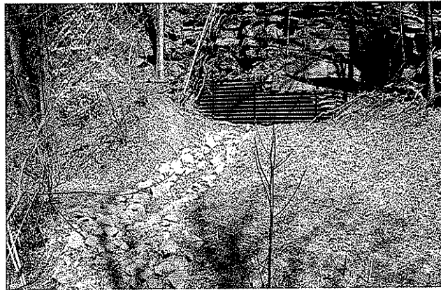
Bat Gate with rip rap channel
