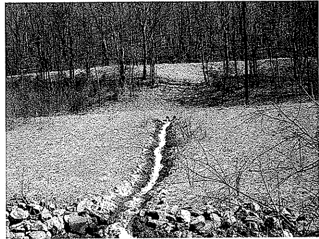
Wet mine seal with rip rap channel
