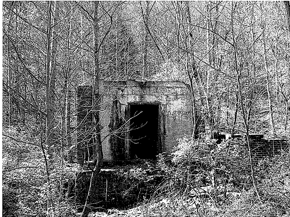
Picture 1 is of one of the remaining abandoned structures.
