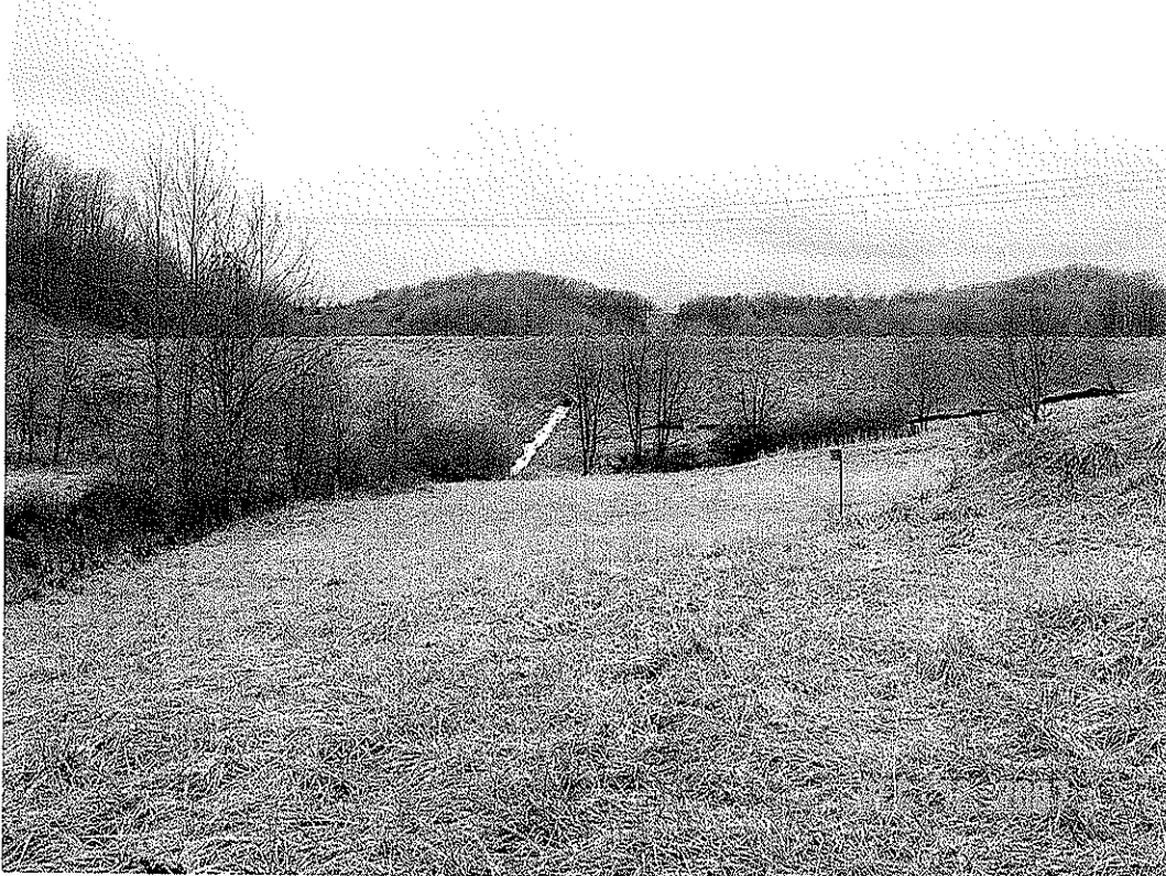
LEMLEY DAM MODIFICATION, MONONGALIA CO., WV
