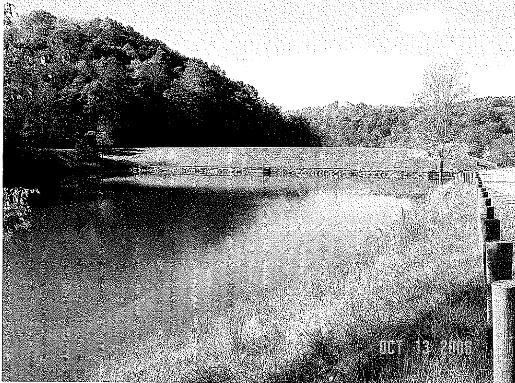
JIMMY LEWIS DAM MODIFICATION, MERCER CO., WV
