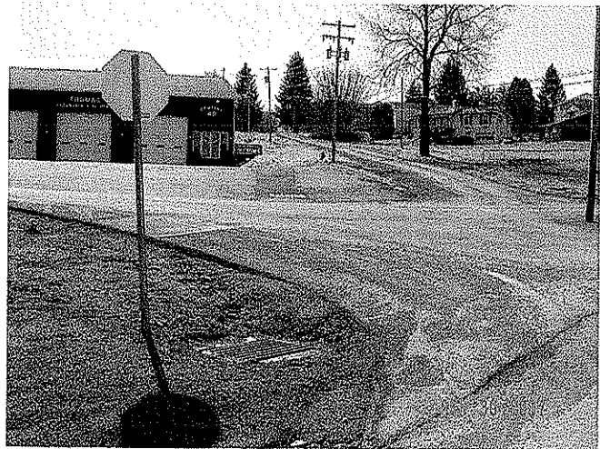
New Storm Drains and Catch Basins
