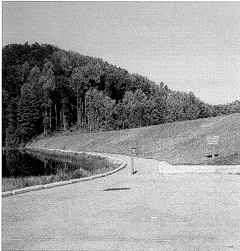
TETER CREEK DAM MODIFICATION, BARBOUR CO., WV
