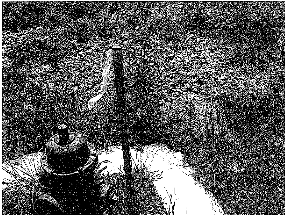
Picture 6 shows a survey point and evidence of buried utilities within the area.
