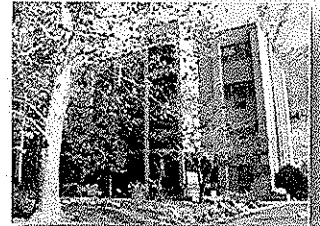
Charleston, West Virginia Office
