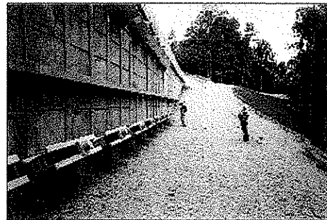
Finished wall with anchors
