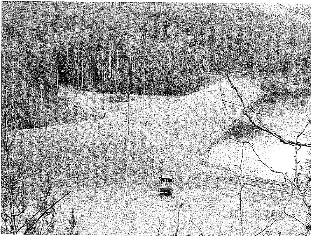
PLUM ORCHARD DAM MODIFICATION, FAYETTE CO., WV
