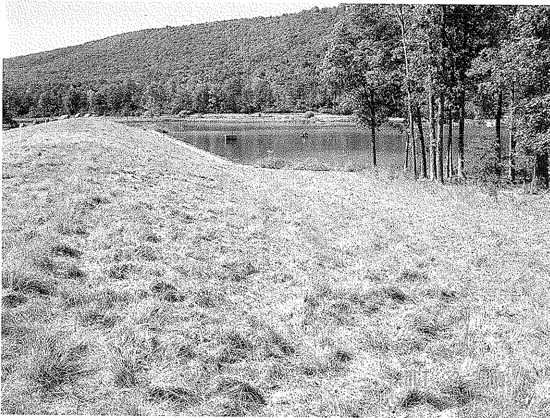
WARDEN LAKE DAM MODIFICATION, HARDY CO., WV
