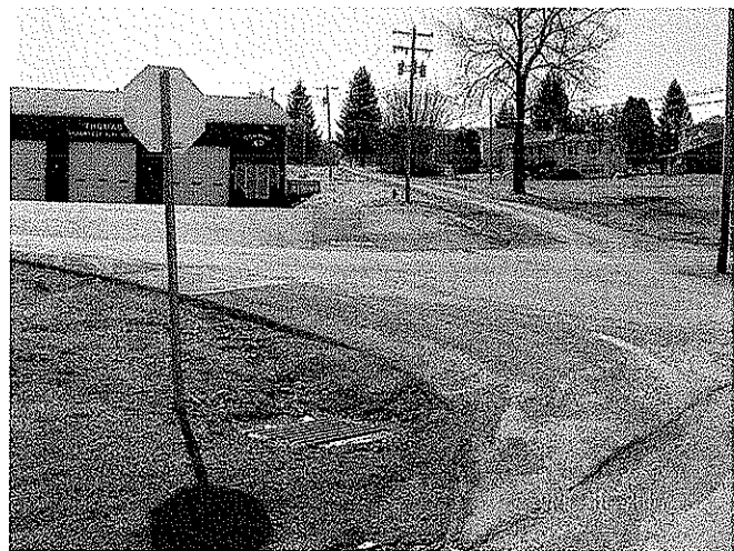
New Storm Drains and Catch Basins
