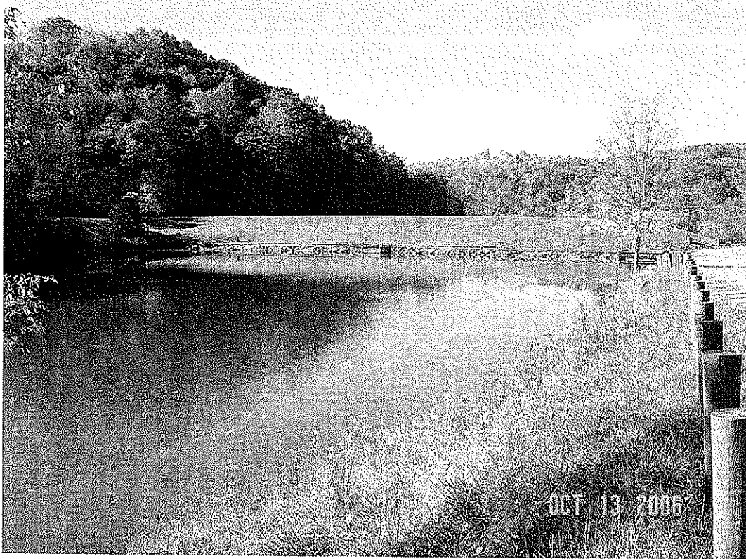
JIMMY LEWIS DAM MODIFICATION, MERCER CO., WV
