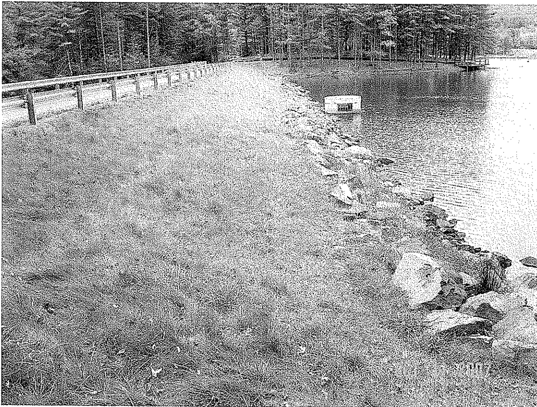
MONCOVE DAM MODIFICATION, MONROE CO., WV
