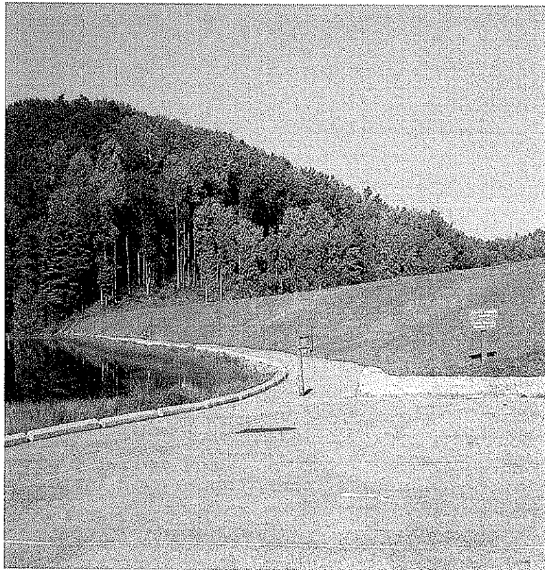
TETER CREEK DAM MODIFICATION, BARBOUR CO., WV
