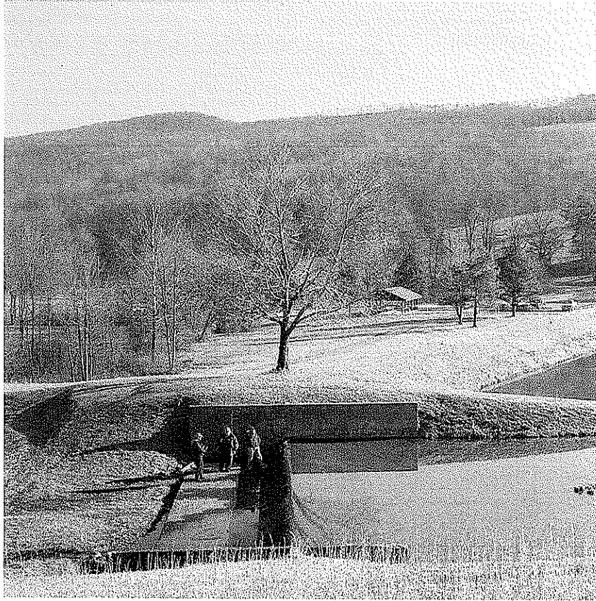
BELINGTON DAM MODIFICATION, BELINGTON, WV
