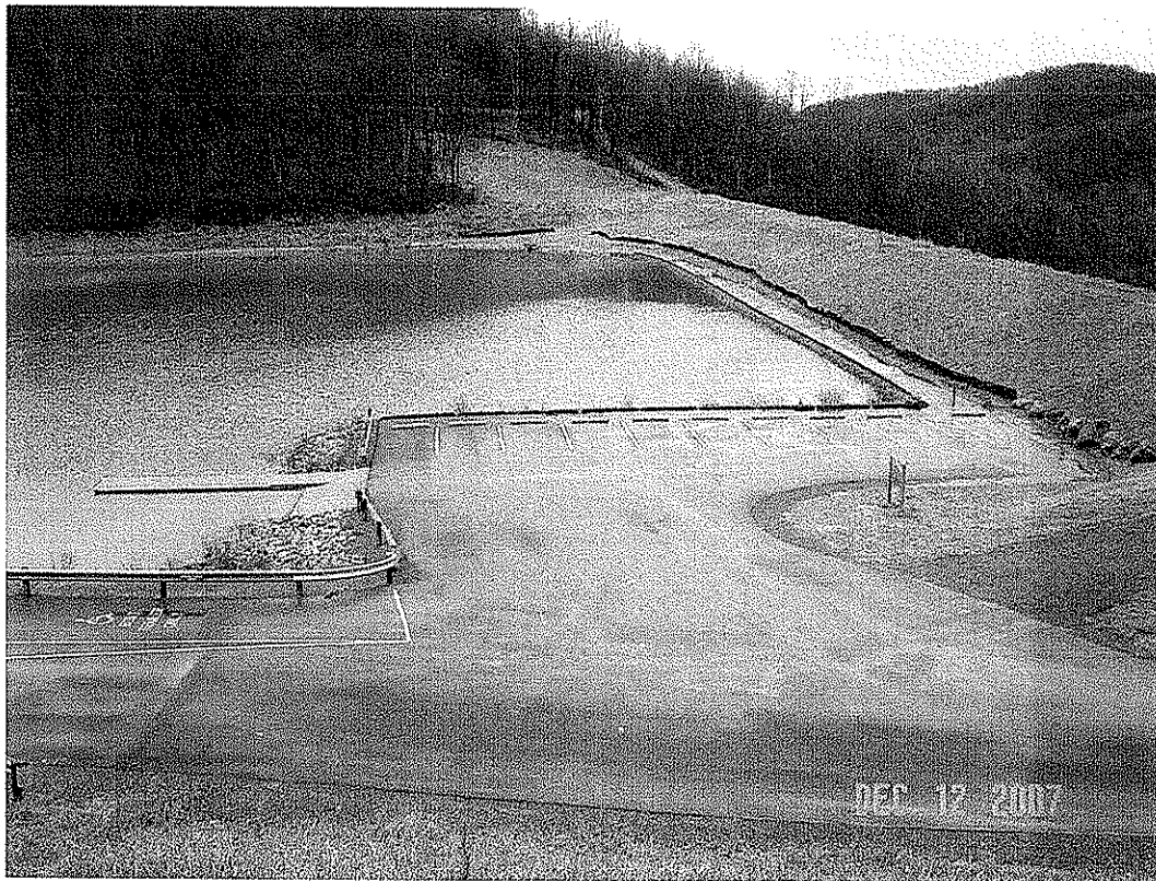
BAILEY DAM MODIFICATION, MONONGALIA CO., WV
