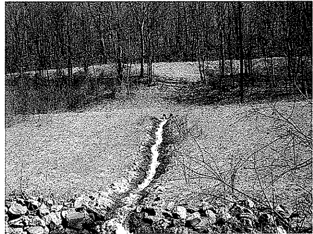
Wet mine seal with rip rap channel
