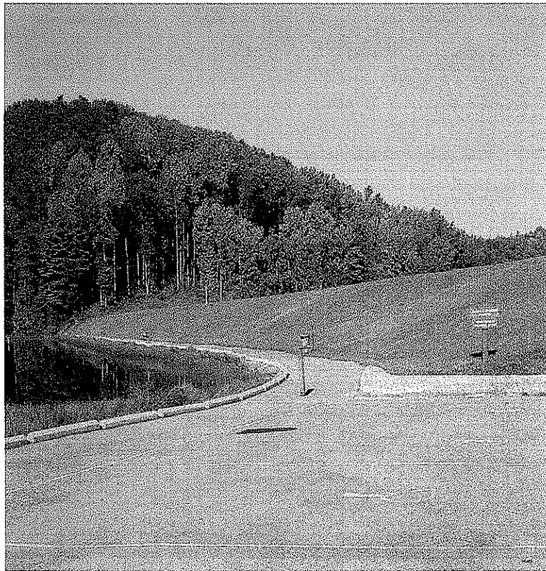
TETER CREEK DAM MODIFICATION, BARBOUR CO., WV
