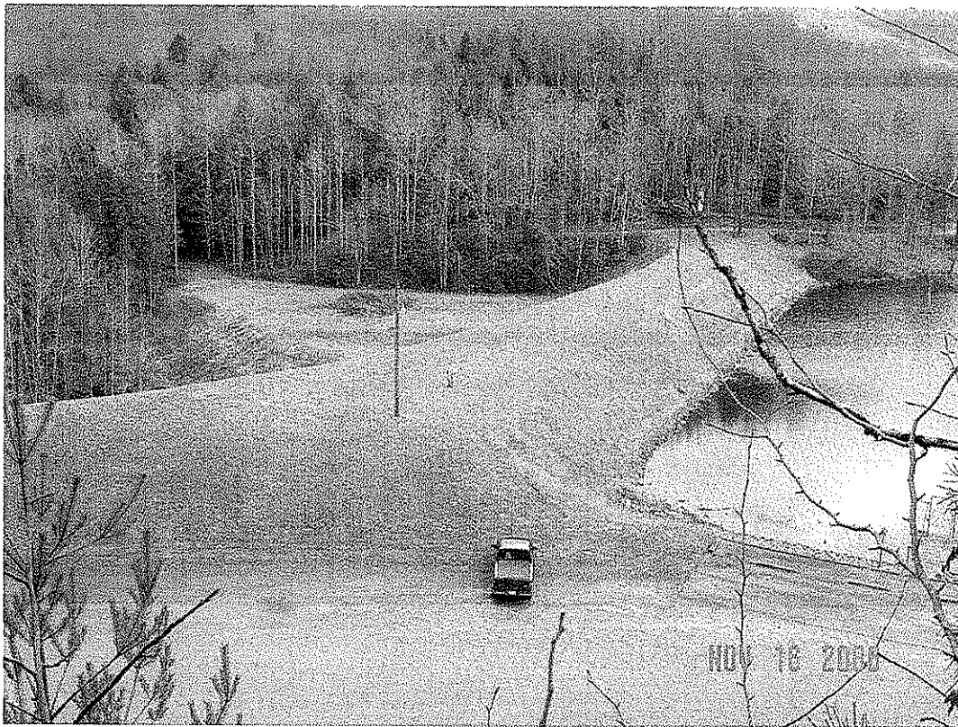
PLUM ORCHARD DAM MODIFICATION, FAYETTE CO., WV
