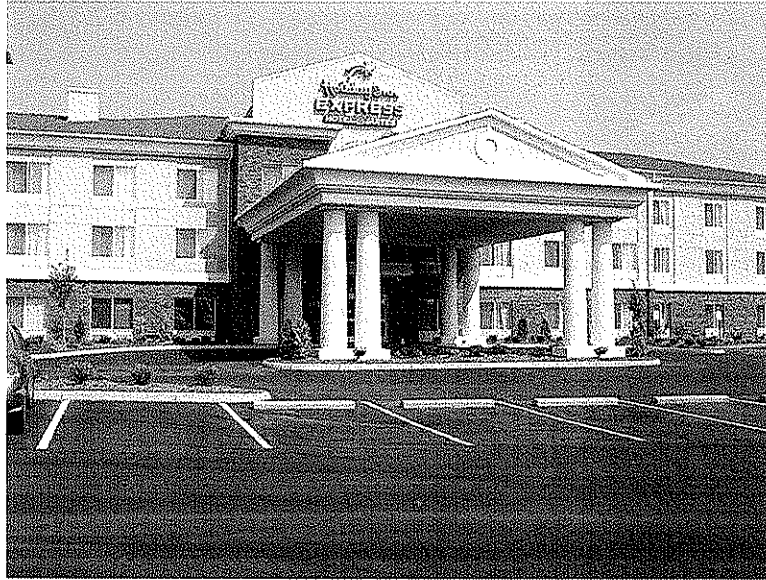
HOLIDAY INN EXPRESS – MINERAL WELLS, WV PROJECT COST UNKNOWN – COMPLETE 2007
