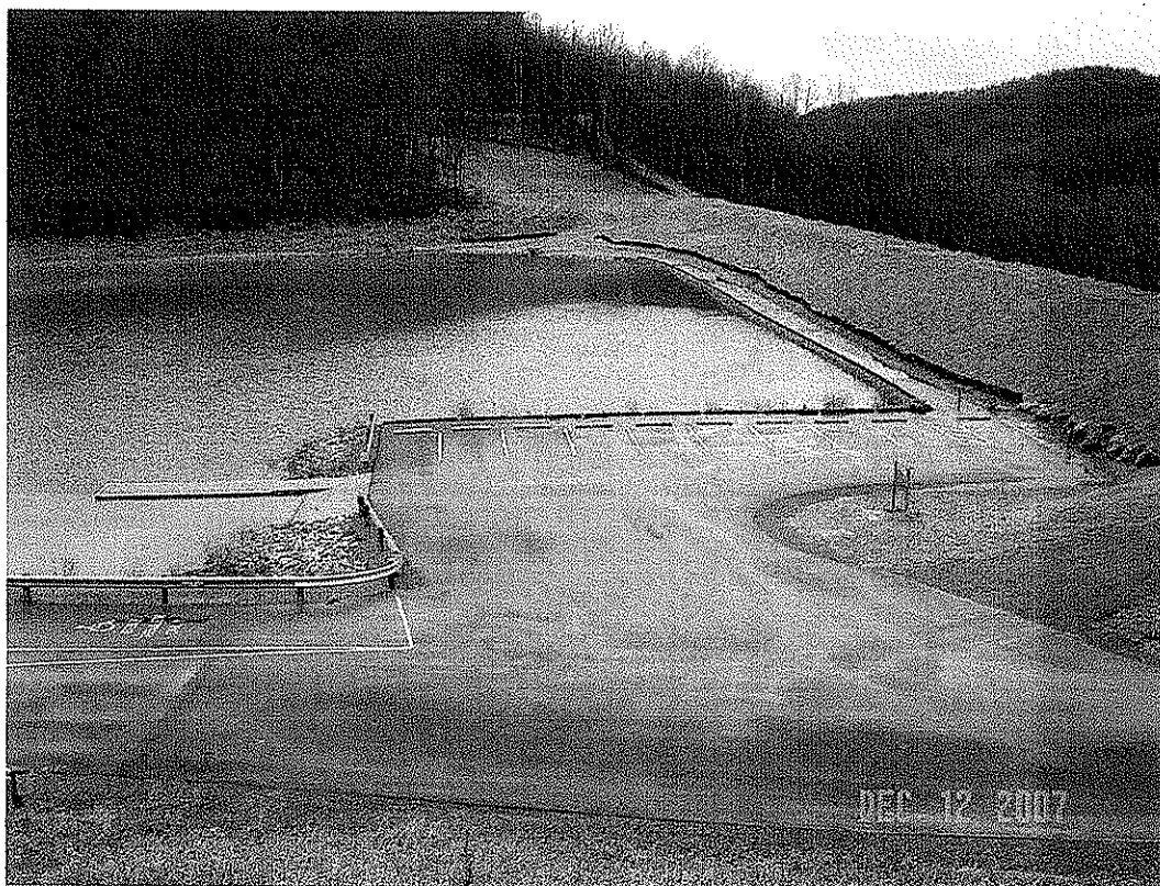
BAILEY DAM MODIFICATION, MONONGALIA CO., WV
