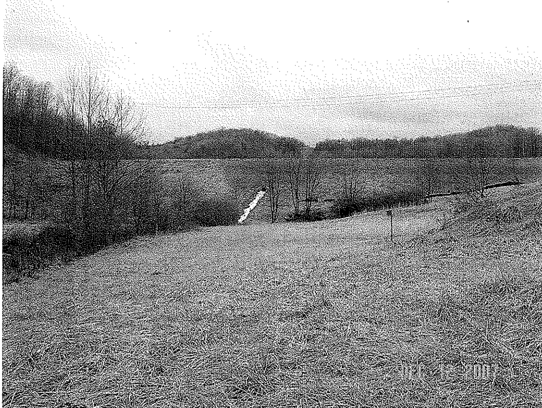
LEMLEY DAM MODIFICATION, MONONGALIA CO., WV
