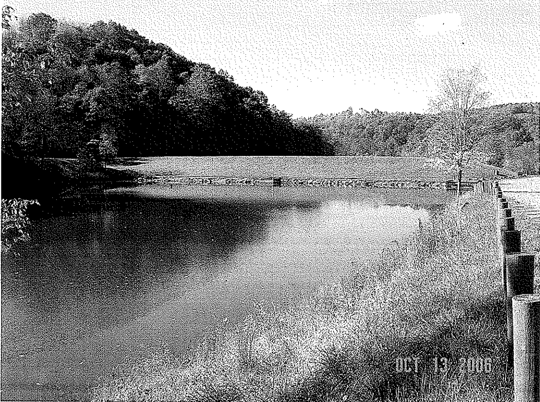
JIMMY LEWIS DAM MODIFICATION, MERCER CO., WV
