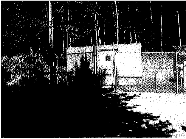
150 GPM Little Sand Run Booster Station
