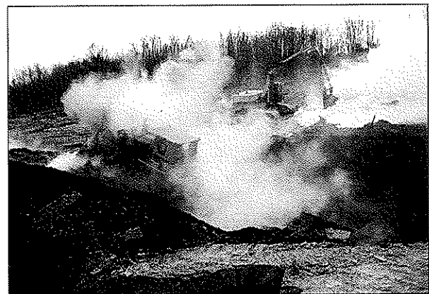
Jamison Burning Refuse Reclamation Project
