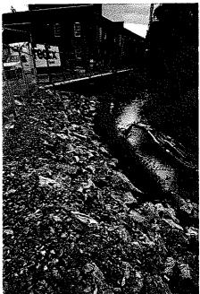
The overall proposed improvements consisted of re-alignment of the stream and the installation of rock vanes to redirect the flow so as to reduce near bank shear stress along the outside bend (previous location of gabion baskets). Other alternatives were investigated; however, concrete and gabion basket walls have been used in the past with a poor success rating.
