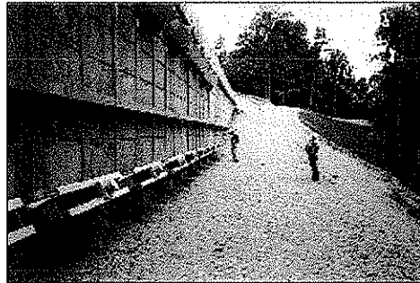
Finished wall with anchors
