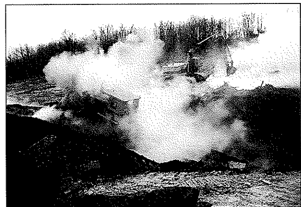
Jamison Burning Refuse Reclamation Project
