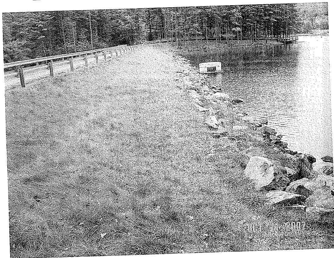
MONCOVE DAM MODIFICATION, MONROE CO., WV
