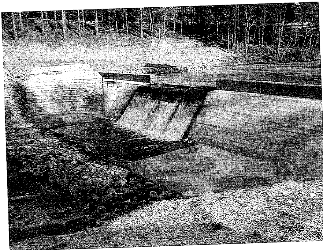
THOMAS DAM MODIFICATION, THOMAS, WV
