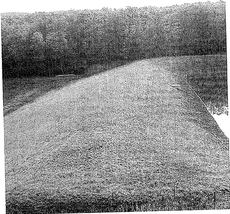
WILSON DAM MODIFICATION, HAMPSHIRE CO., WV
