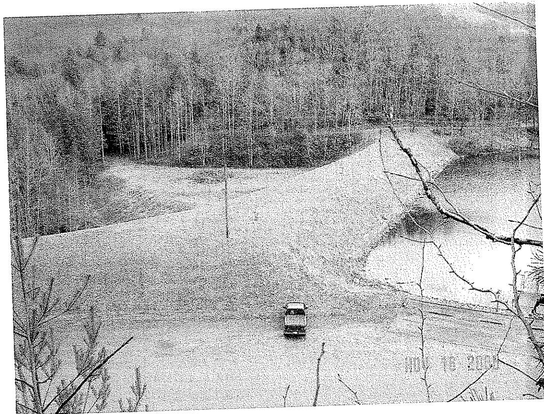
PLUM ORCHARD DAM MODIFICATION, FAYETTE CO., WV
