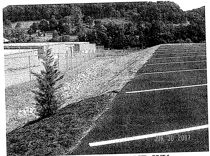
MT. VERNON BAPTIST PARKING LOT EXPANSION – HURRICANE, WV PROJECT COST $ 50,000 – COMPLETE 2007
