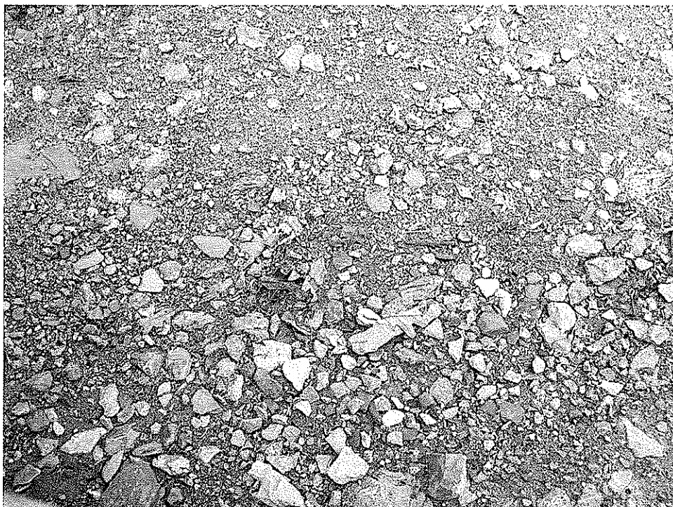
Additional evidence of coal refuse on the site
