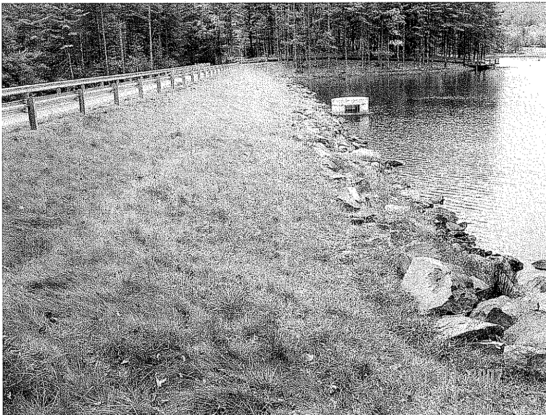
MONCOVE DAM MODIFICATION, MONROE CO., WV
