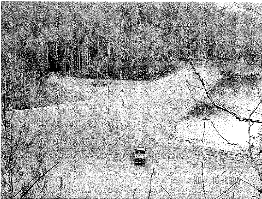
PLUM ORCHARD DAM MODIFICATION, FAYETTE CO., WV
