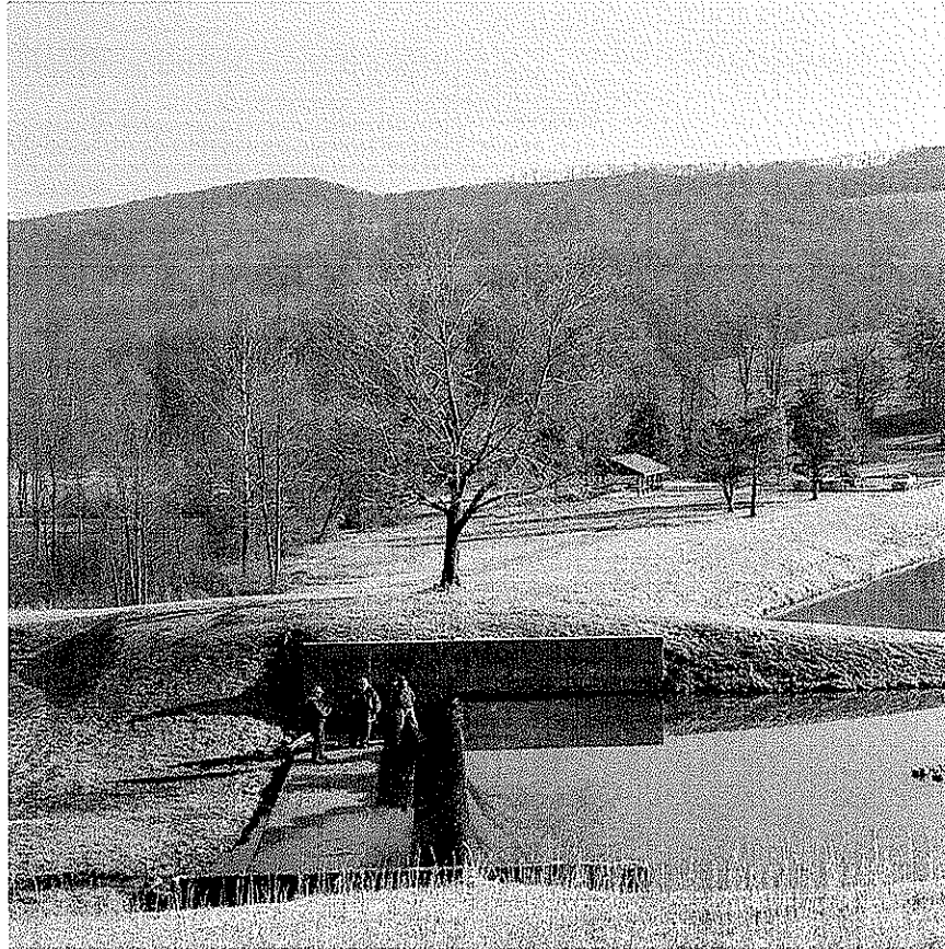
BELINGTON DAM MODIFICATION, BELINGTON, WV
