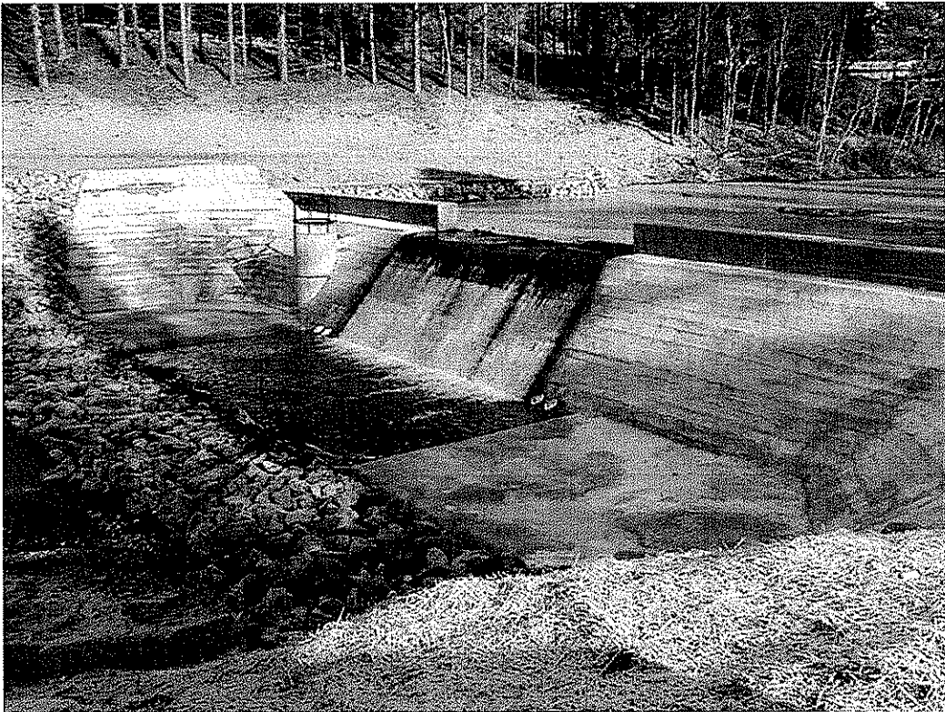
THOMAS DAM MODIFICATION, THOMAS, WV
