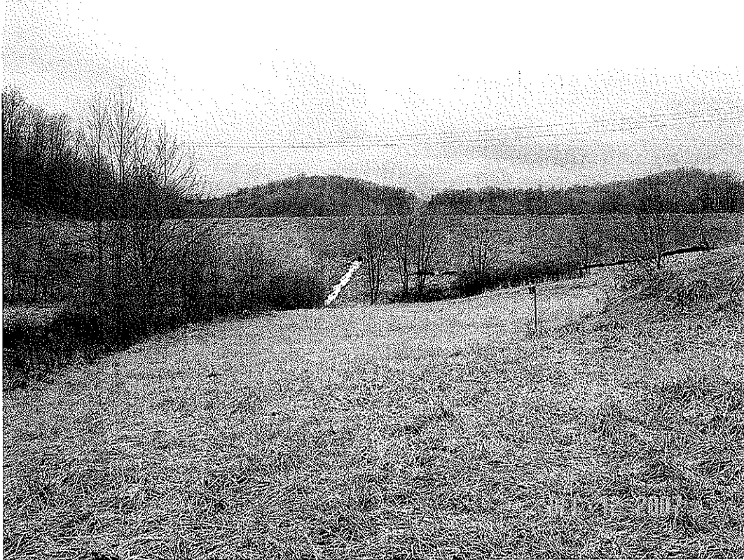
LEMLEY DAM MODIFICATION, MONONGALIA CO., WV
