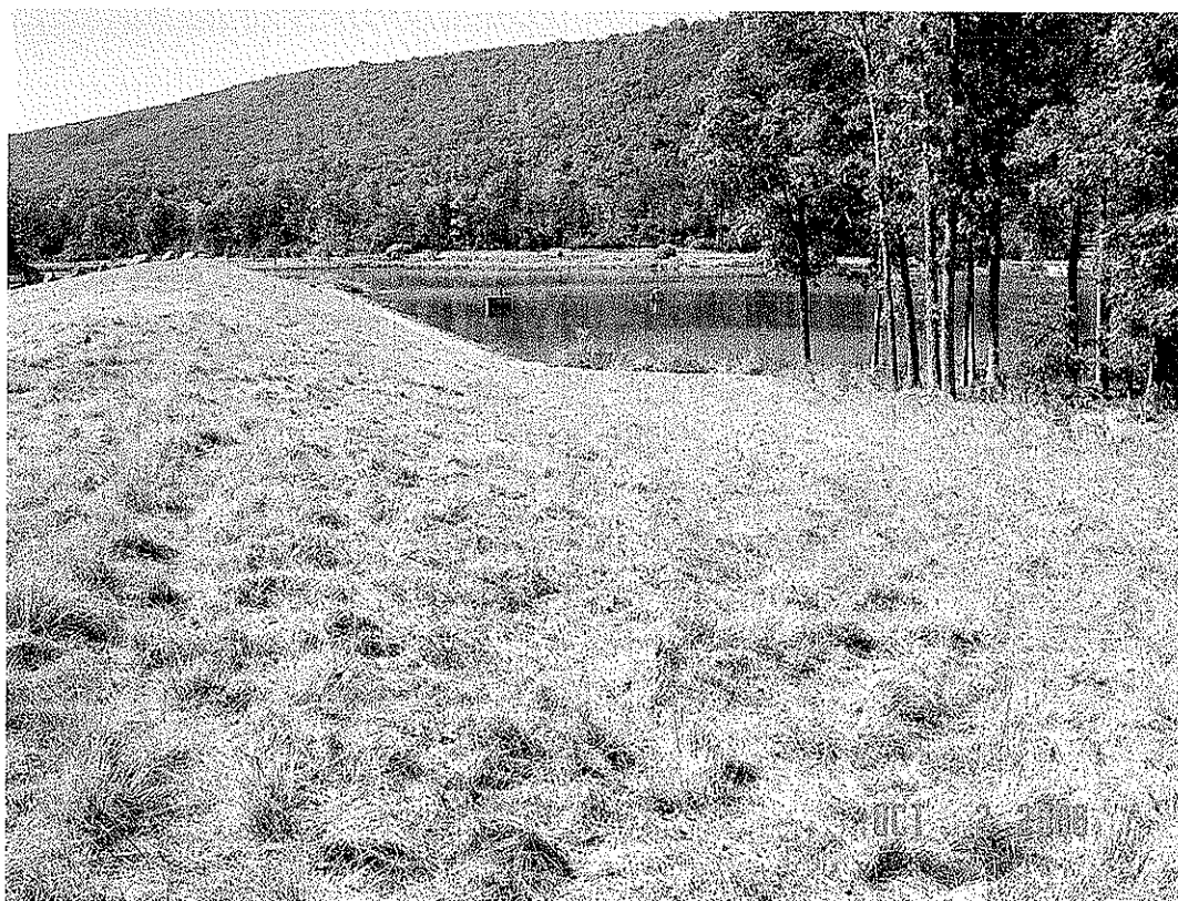
WARDEN LAKE DAM MODIFICATION, HARDY CO., WV
