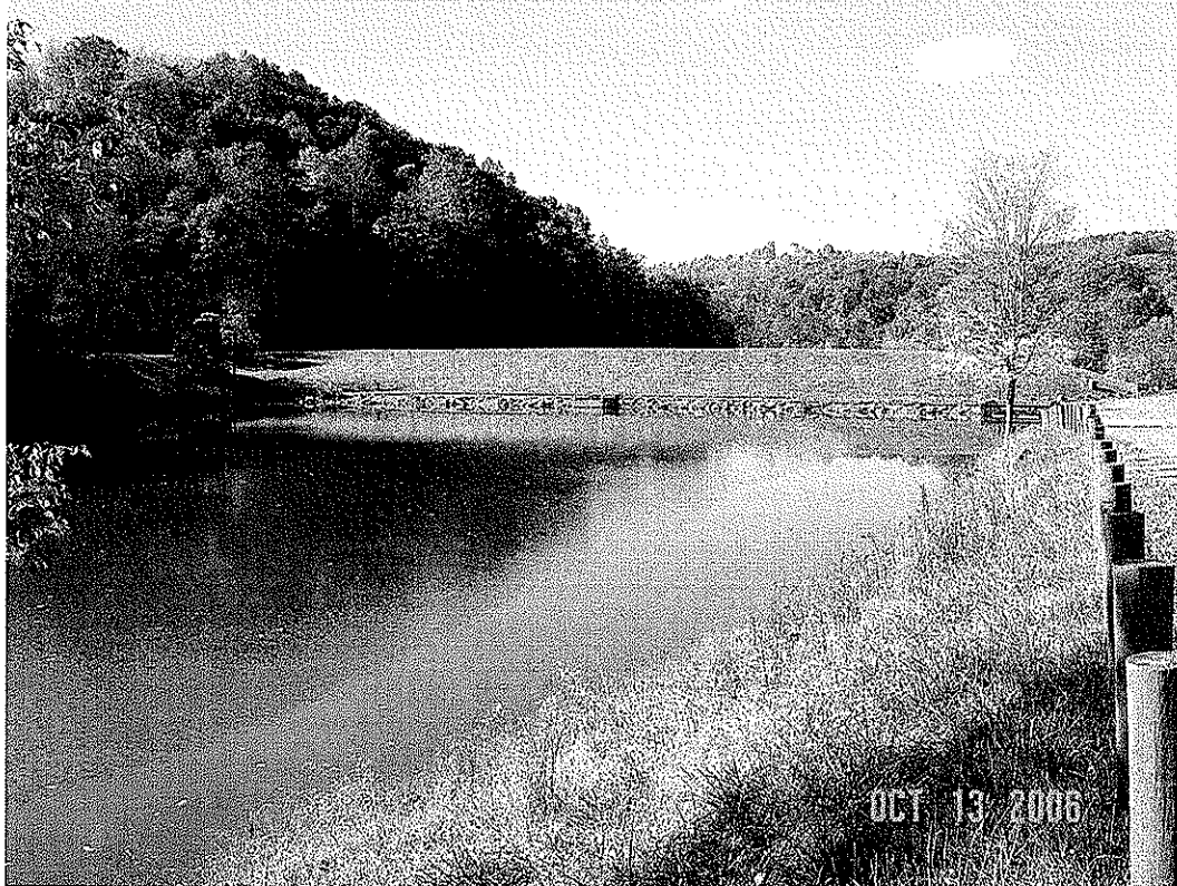
JIMMY LEWIS DAM MODIFICATION, MERCER CO., WV
