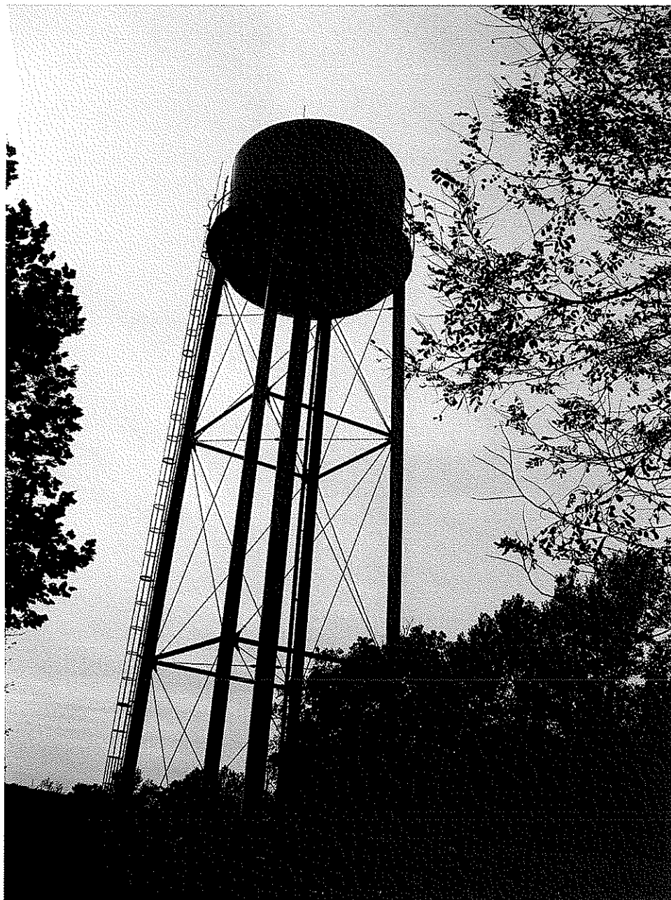
Water storage tank located above the site
