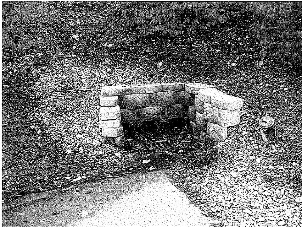
The drop inlet in the driveway of 3961 East Lake Drive
