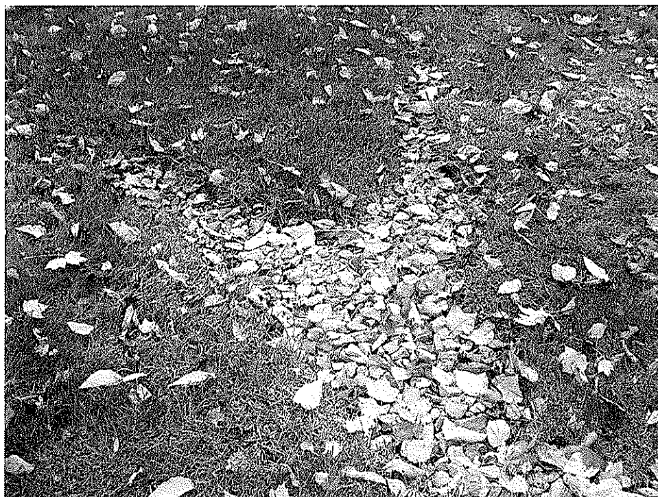
French drain installed behind 3959 East Lake Drive
