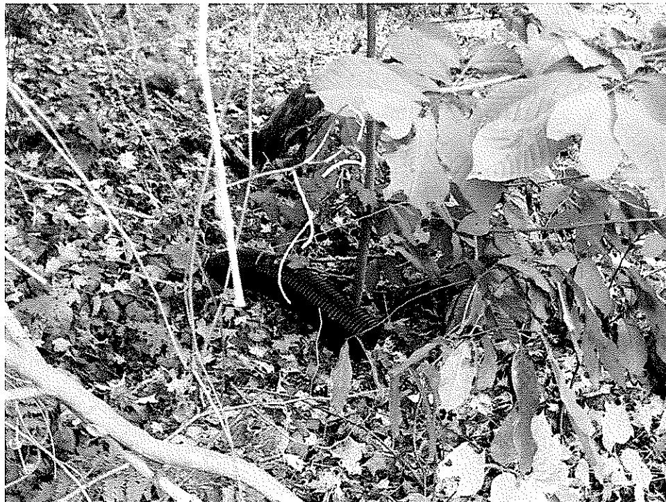
Flexible drain pipe installed near the collapsed portal
